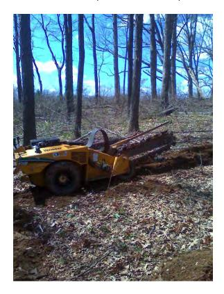
The trencher used to sever belowground roots sits within the midstory removal treatment at our drier site, prior to planting in the spring of 2009.
